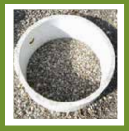
Figure 4: Pipe Installed Into Media
