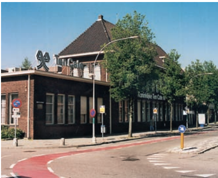
Koninklijke Ten Cate nv, corporate headquarters in Almelo, the Netherlands.
